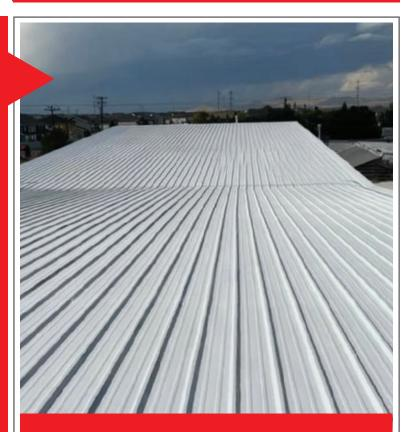
The key difference is in the design and application – standing seam roofs take full advantage of having concealed fasteners. A standing seam system consists of wide, relatively flat metal panels that have vertical legs (or ribs) on each end.
